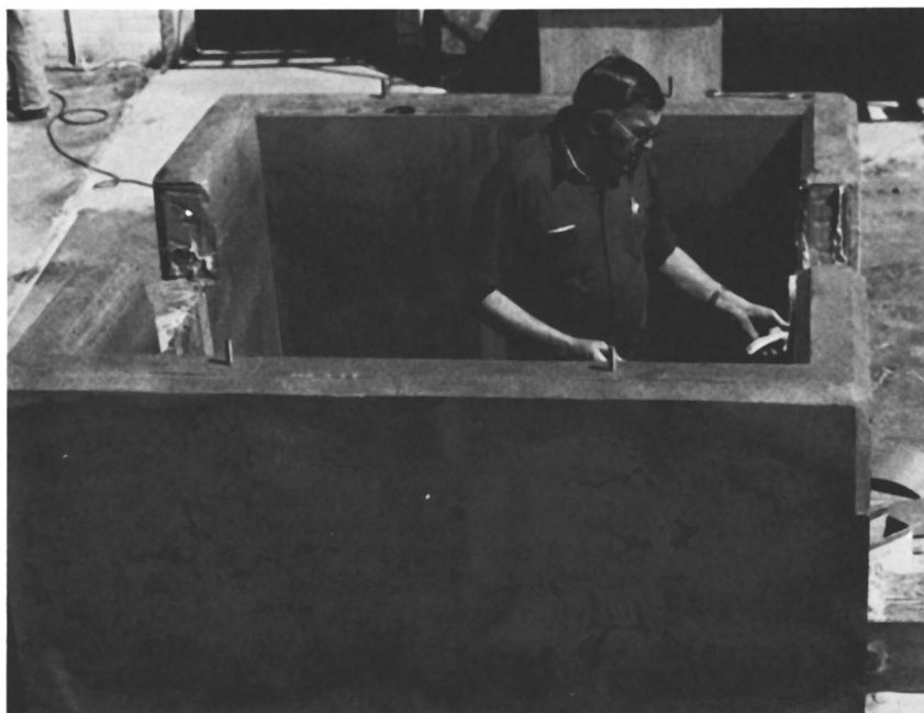
Figure 1. Sulfur concrete sump for installation in the zinc electrolyte pumping circuit.
