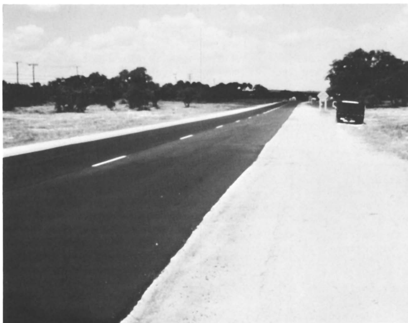
Figure 1. Completed Sulphlex pavement (right-hand lane) on Loop 1604, August 1980.
