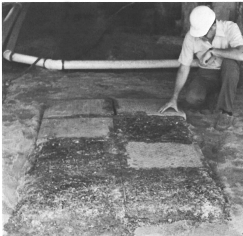
Figure 2. Sulfur concrete and control portland cement concrete (4-test sections each) in the floor area of the electrolytic zinc refinery. After 28 months, no corrosive attack is seen on the sulfur concrete sections, although the control samples were severely attacked.
